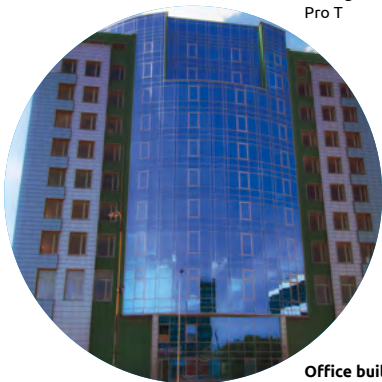
Office building, Saint Petersburg, Russia Pilkington Suncool™ -R Blue 50/25 Pro T
